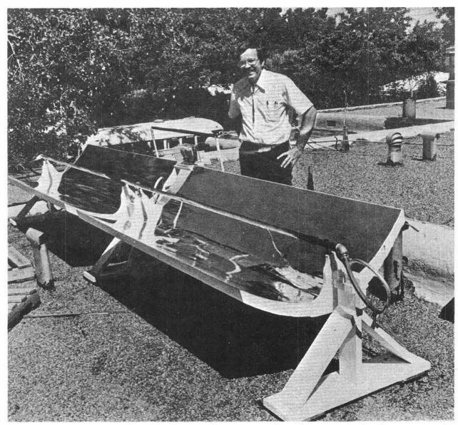
UP TO THE SUN. Bob Stromberg (5714) uses solar energy to heat hot water for his home. Sensor he designed and built tracks the sun and keeps rooftop parabolic collector troughs properly oriented. Entire system was built in about five months (nights and weekends), mostly from surplus materials.
